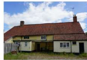
Rear elevation with 20 th Century extensions
