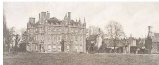
East Elevation, Cockfield Hall 1937
