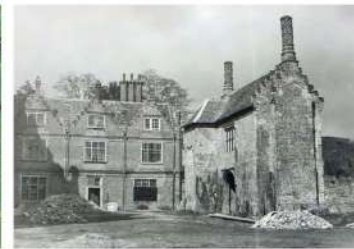
1943 photograph of the north wing and gatehouse with piles of rubble and boarded up windows, indicating repair and rebuilding work following bombing in World War II (photographer T.E. Legg, Historic England Rail Box Collection, Card reference no. S665,079).
