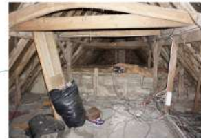
View looking through the rused aisle framing with late 17 th /18 th century rebuilt purlin roof at the far end
