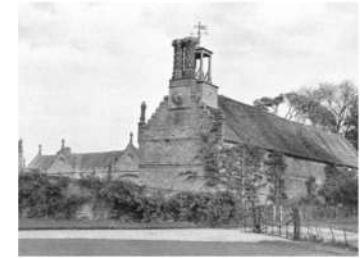
South East Elevation, Clocktower 1924
