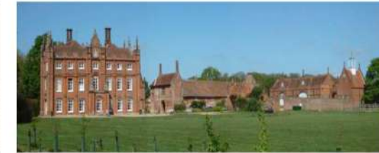
East Elevation, Cockfield Hall 2015
