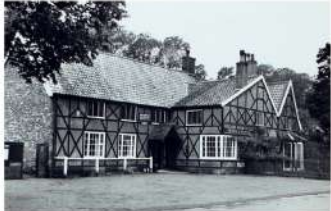
1939 photograph of the Griffin, showing rebuilt south gable and straightened roof pitch of the range on the front of the building. (England's Places)
